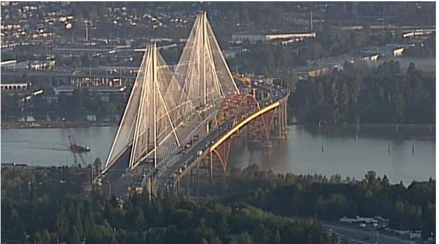
New Port Mann Bridge adjacent to the old bridge
